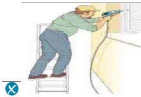
Incorrect – steps side on to work activity
