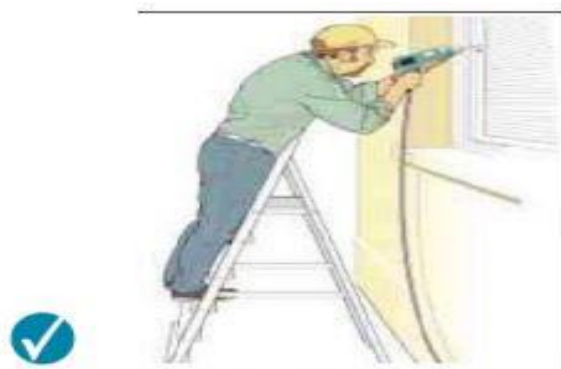
Correct – steps facing work activity
